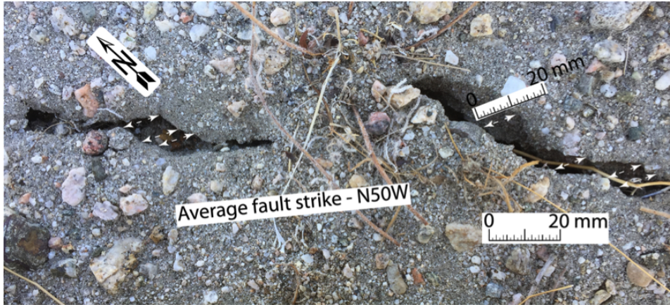
Figure 5. Example of an echelon surface rupture associated with a creep event showing the small dilational steps used to measure displacement. Displacement in this example is estimated at 11 mm.
